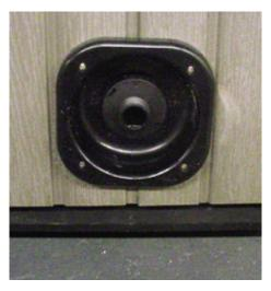
Figure 20. Cabinet mounted drain valve
