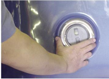
Figure 11. Rotating an adjustable jet
