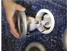
To replace jets, insert the jet in the jet well and push and rotate it clockwise until you feel it snap into position. When the jet face can be rotated freely, it is properly seated.
