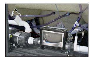
After the spa has been placed on an approved surface and has been correctly wired by a licensed electrician, inspect all plumbing connections in the equipment area of your spa. Ensure that these connections are secure and that they did not loosen during shipment.
