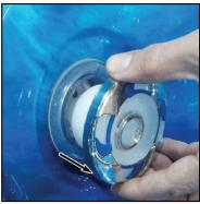
Note: have the jets turned off when removing jet inserts, it will be easier to remove when there is no water flow through it.
