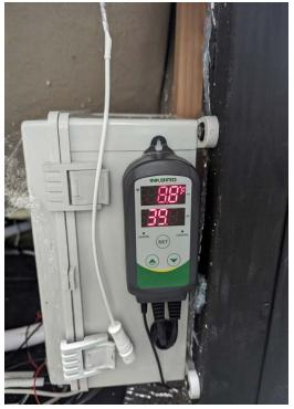
Select your lowest temperature, use the up or down arrows to adjust set point, the lowest the unit can support is 39F°. Once set press "set" to save the adjustment a HD will appear after a successful temperature adjustment.
